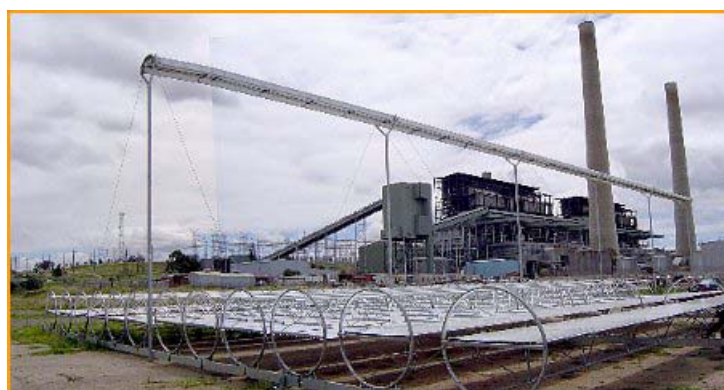
Fig. 3. Fresnel solar field in Australia Source “Solar Heat and Power Europe” [9]
